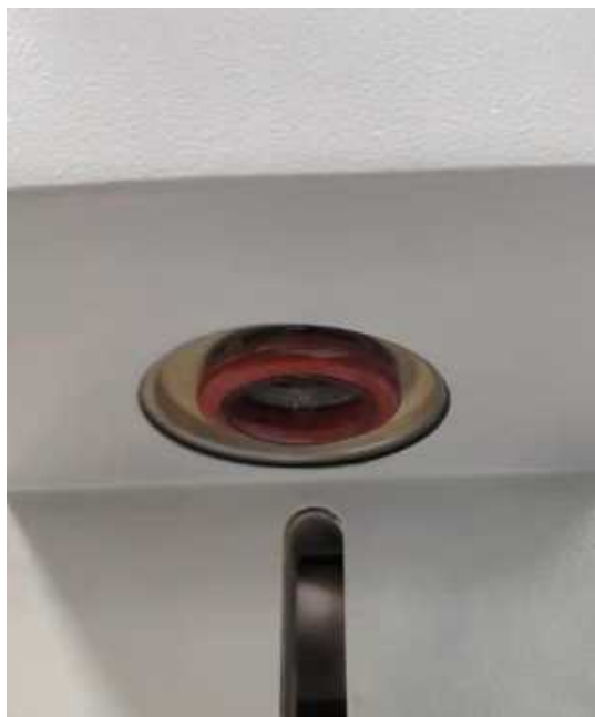
Figure 3-17 Sealing ring at the bottom
