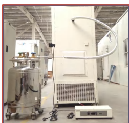
LN 2 /CO 2 backup system
